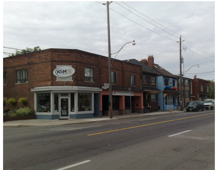
Fig. 1.11: Buildings are typically two storeys in height.
