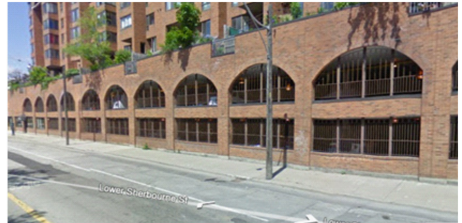
Fig. 2.14: Parking Garage, Lower Sherbourne Street Source: Google Image
