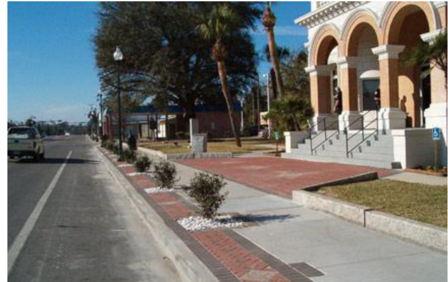
Fig. 2.39: Paved sidewalk with strip of interlocking brick. Source: Clough Harbour & Associates, 2009.
